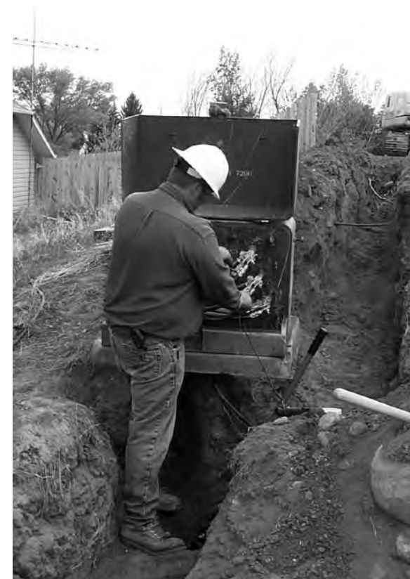
Underground line replacement
