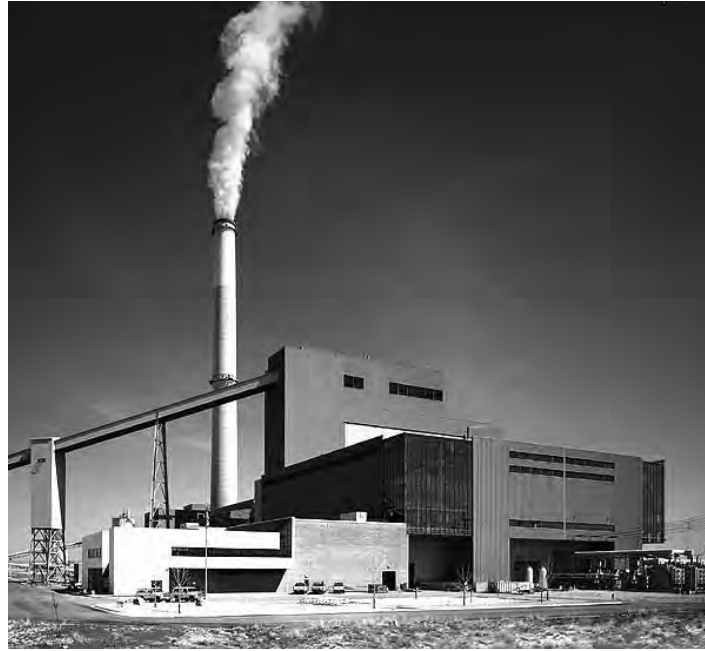
Bonanza Power Plant
