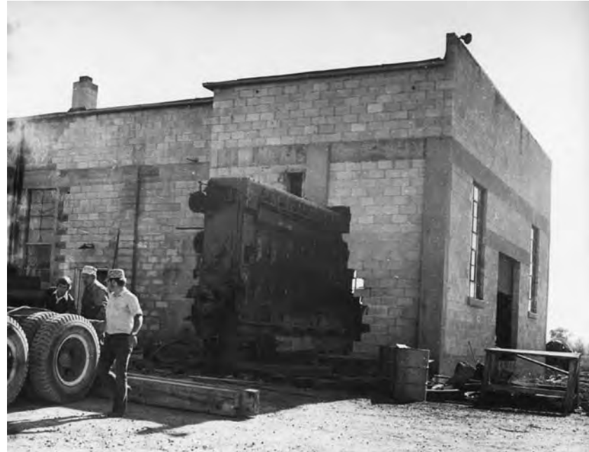
Rangely generator move
