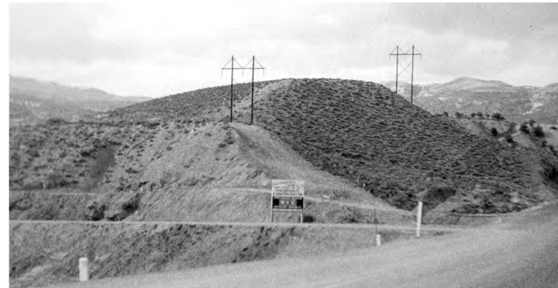
Moon Lake's 138 kV transmission line serves Dutch John and Flaming Gorge Dam.
