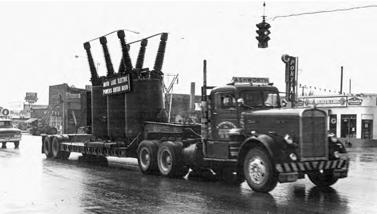
Circuit breakers for the Southwest Rangely substation
