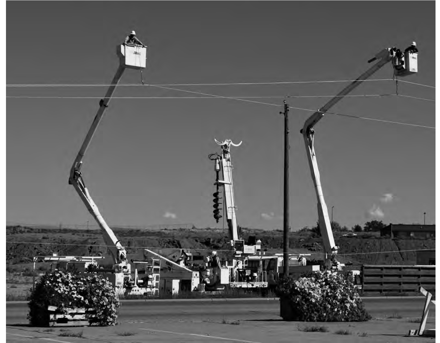
Tyler Lisonbee, Gary Nelson, Brett Miles, and Robert Richens replace a pole hit by a truck, 2012.
