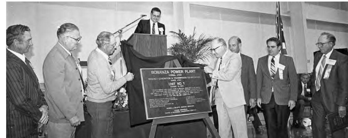
The Bonanza Power Plant was dedicated in 1985.
