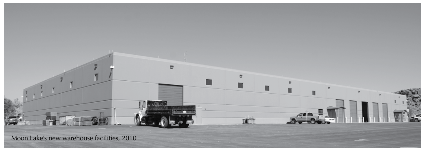
Moon Lake's new Roosevelt office and warehouse complex, 2010
